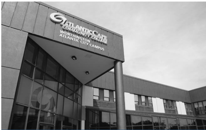
WORTHINGTON ATLANTIC CITY CAMPUS 1535 Bacharach Blvd., Atlantic City
